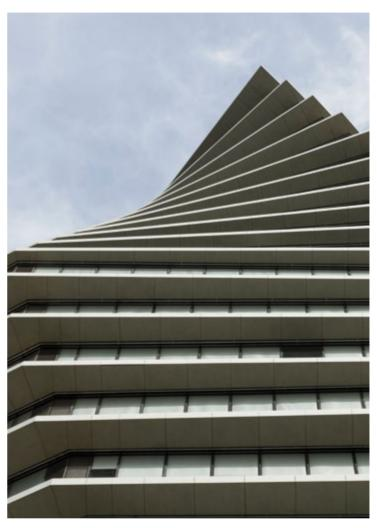
On the intermediate floors, the broken perimeter of the concrete slabs is clad with panels 12 millimetres thick and up to two metres wide which, thanks to minutely accurate cutting, define the vertexes and edges exactly to create an image of perfection.
