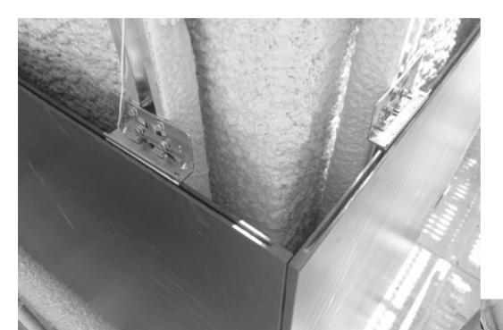
Dekton® has the certification for ventilated façades according to ETA 14/0413 and BBA 16/5346 for 12mm and 20mm thicknesses, although it can be used for other non-certified thicknesses.
