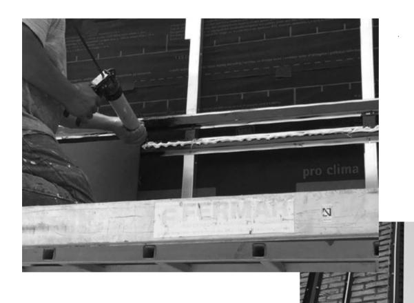
Fixing with chemical anchoring on profiles.
