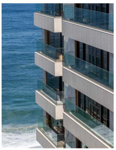
Di Filippo Arquitectura chose Dekton® by Cosentino for the façade for various reasons: it represented just 50% of the permitted load for the material, it can be manufactured in large format, bespoke slabs (3.2 m x 1.44 m), the precision cutting of pieces, its optimal performance against sand and saltwater erosion from the beach, and its other exceptional qualities such as its high resistance to ultraviolet rays, its colour stability and high resistance to stains.
