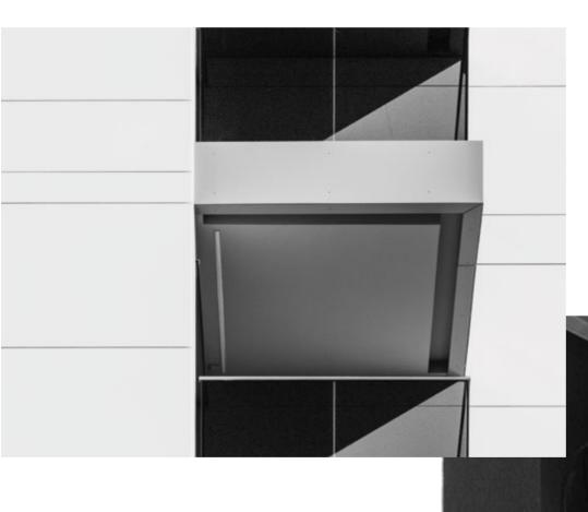
This solution creates an almost hermetic ventilated chamber, due to the continuity of the supporting profile itself. Dekton® has the certification for ventilated façades according to ETA 14/0413 and BBA 16/5346 for 12mm and 20mm thicknesses, although it can also be used with 30mm.
