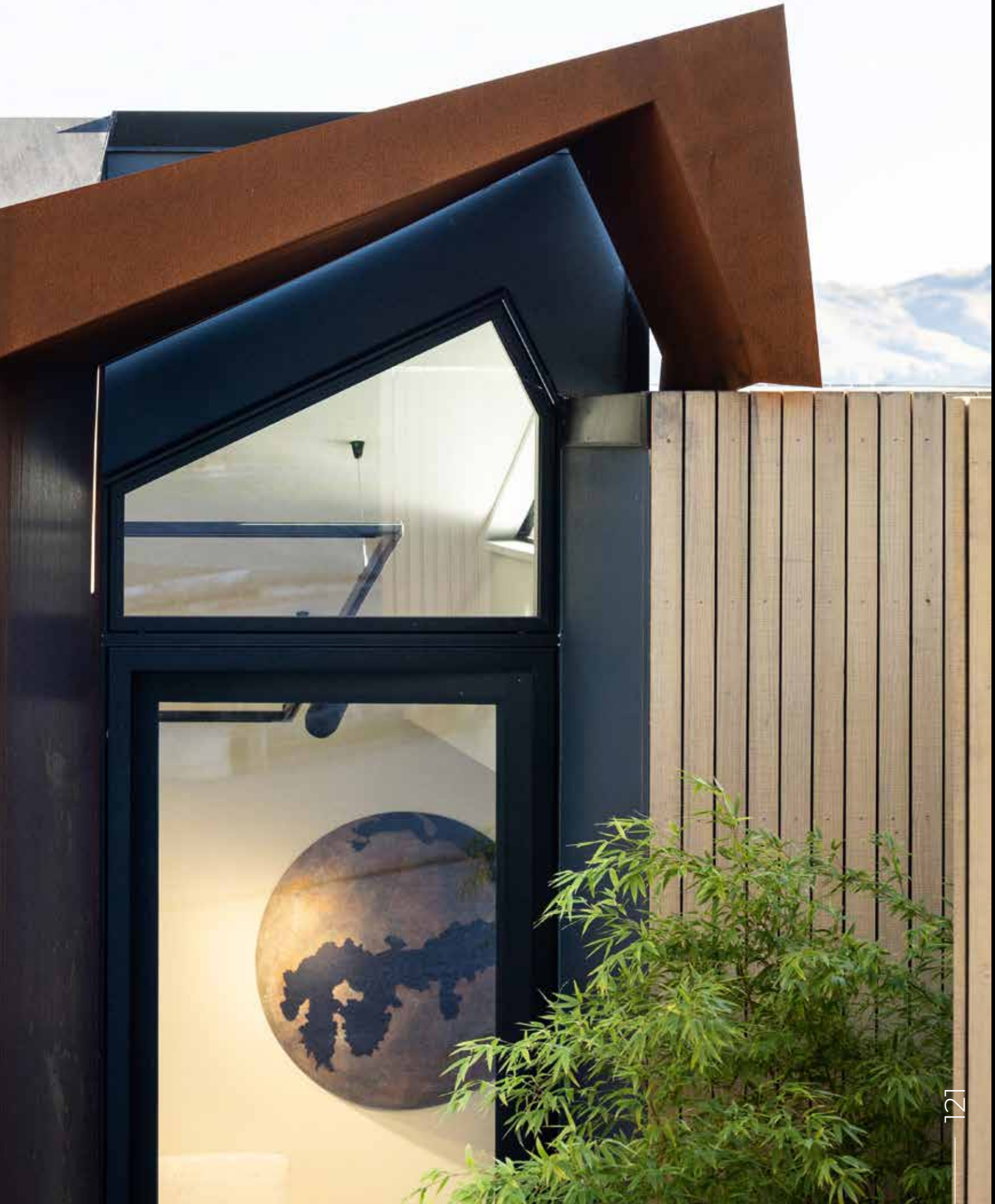
Private residence, Christchurch (New Zealand) Ventilated facade: Zaha Stone and Basalt Black Designed by: MC Architecture Studio Ltd Image: Clinton Lloyd
